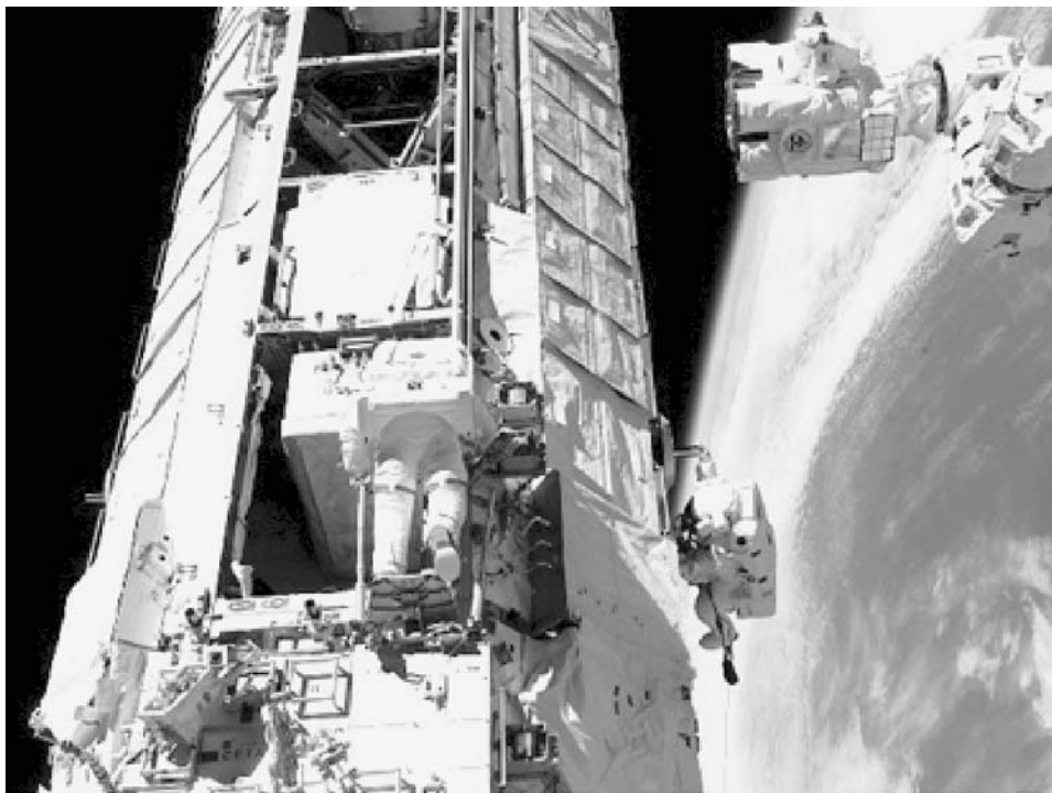
Figure 2. Astronauts of STS 113 install the 13.7 m long P1 truss on the International Space Station in November 2002. In the future, this kind of large-scale construction experience will pave the way for the building of large astronomical facilities, and other pieces of scientific infrastructure, in space (NASA).
